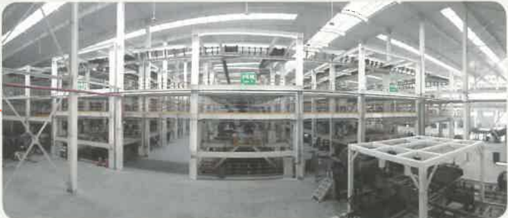
Threading, Air Pressure Test, and Anti-rust Treatment
